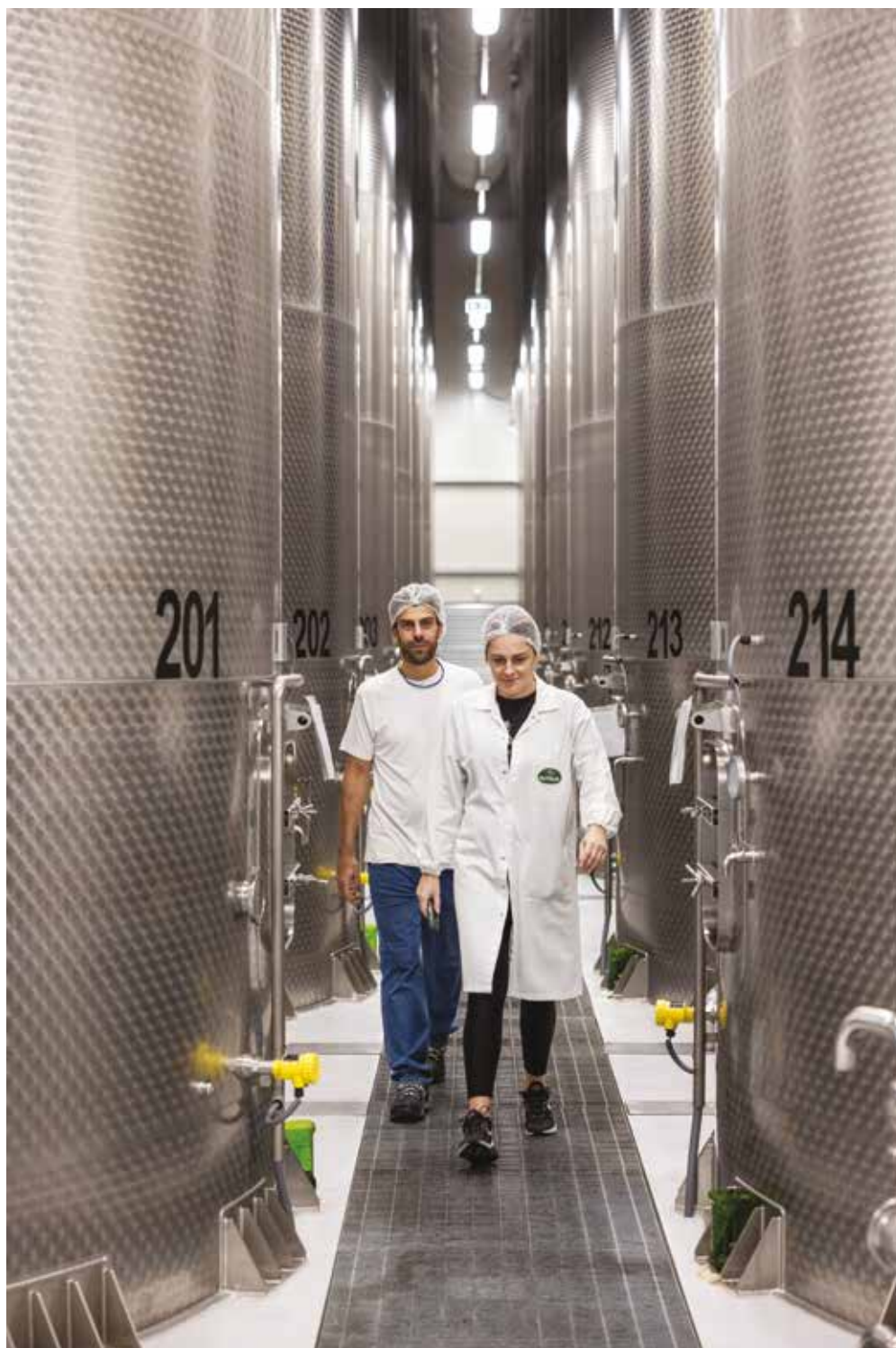
Warehouse B1: tanks in an air-conditioned environment
